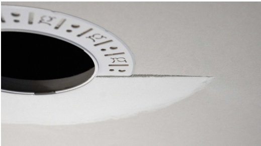
Partially finished mud ring, showing cross-section detail.
