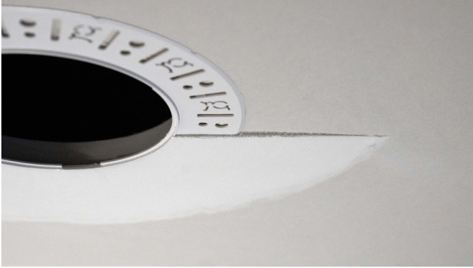
Partially finished mud ring, showing cross-section detail.
